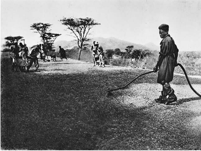
FIGURE 8.2. Application of bitumen to the road surface following the conquest of Ethiopia, ca. 1938. Source: Società Anònima Puricelli Strade e Cave, Lavori in A.O.I. (Milan: Società Anònima Puricelli, 1938). The Wolfsonian–Florida International University, Miami Beach, Florida, the Mitchell Wolfson Jr. Collection, 84.2.300. Photo: David Almeida.
