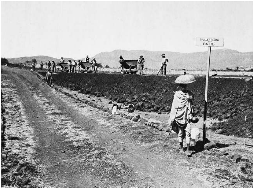
FIGURE 8.3. New Italian road under construction in Ethiopia alongside a “mule track,” ca. 1938. Source: Società Anònima Puricelli Strade e Cave, Lavori in A.O.I. (Milan: Società Anònima Puricelli, 1938). The Wolfsonian–Florida International University, Miami Beach, Florida, the Mitchell Wolfson Jr. Collection, 84.2.300. Photo: David Almeida.
