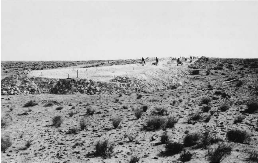
FIGURE 7.3. Preparation of the roadbed in Libya, 1937. Source: La strada litoranea della Libia (Verona: Mondadori, 1937). The Wolfsonian–Florida International University, Miami Beach, Florida, the Mitchell Wolfson Jr. Collection, 84.2.427. Photo: Lynton Gardiner.
